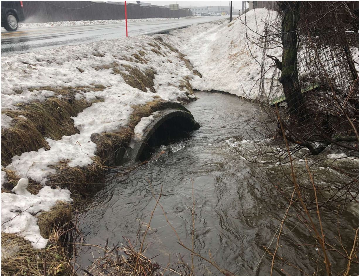
Figur 7. Kulvert 5 under fv 43.
